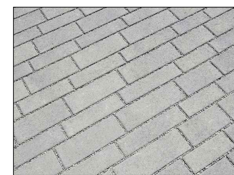
PERMEABLE PAVERS AQUALINA BY ANGELUS BLOCK INC. WITH ROCK CHIPS INSTALLED IN THE PAVER JOINTS TO ALLOW WATER TO FLOW INTO THE BASE UNDERNEATH THE PAVERS
